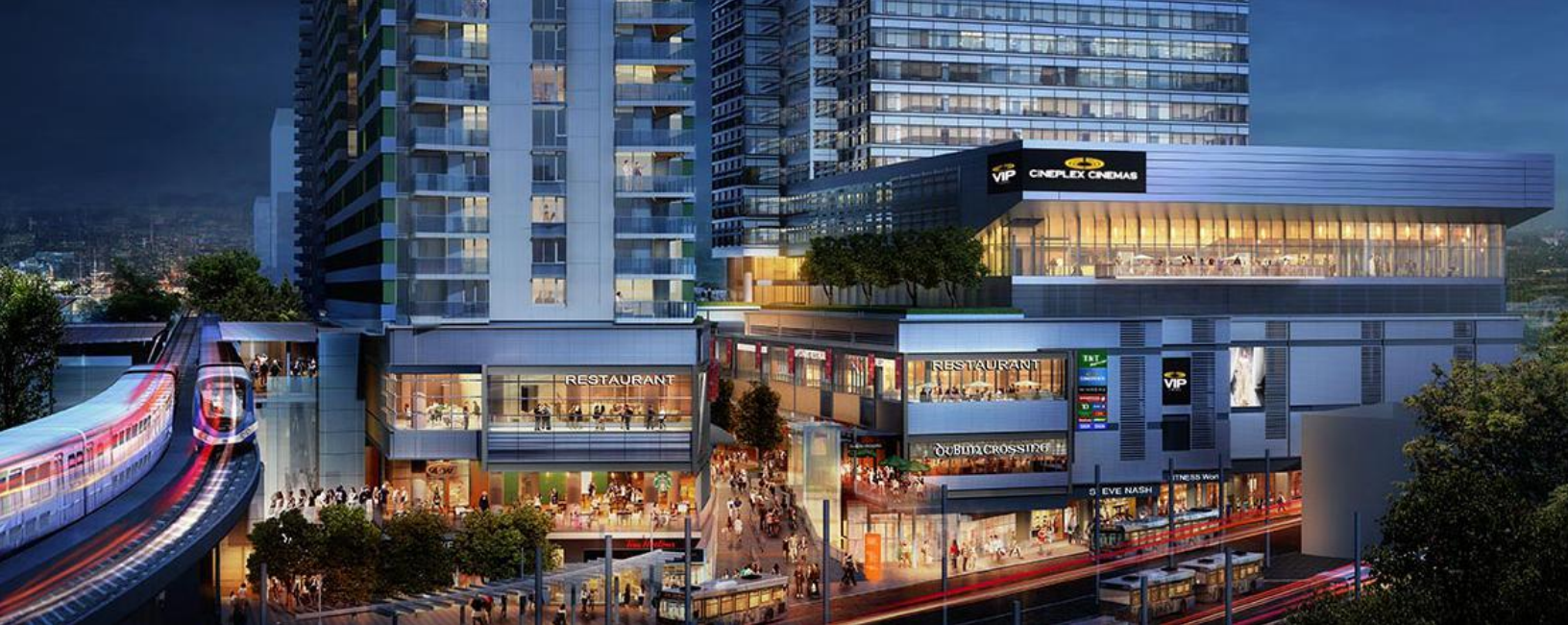
Marine Gateway Transit Oriented Community (source: PCI Group)
